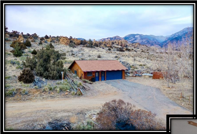
Detached Garage with Office Bunkhouse
