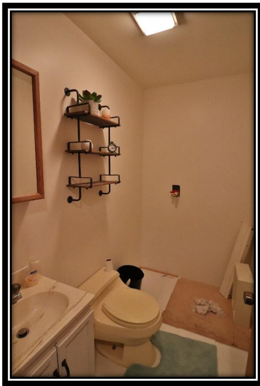
Unfinished Bathroom in Loft
