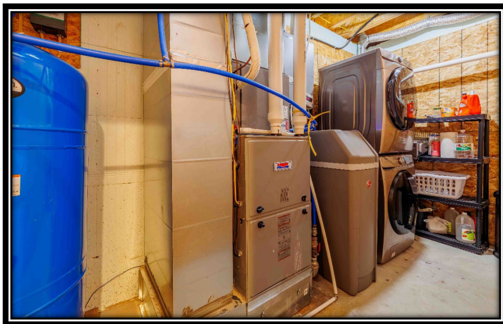
Laundry Utility Room
