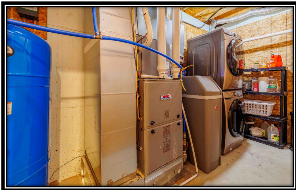
Laundry Utility Room
