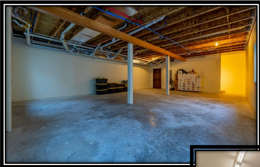
Basement Textured/Painted Walls
