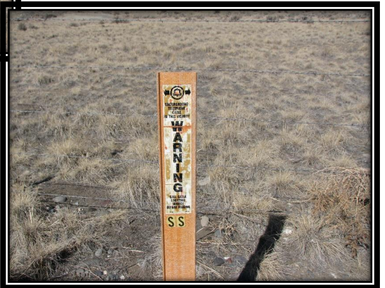
Underground Cable In the Vicinity
