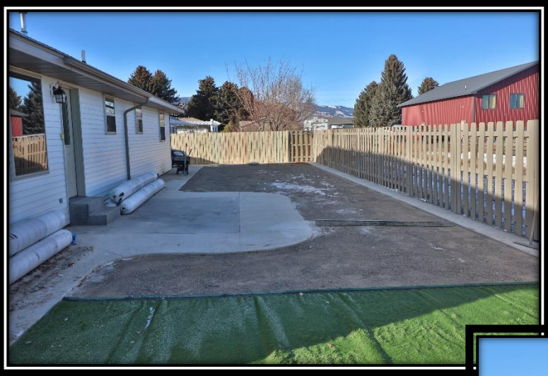
Back Yard Artificial Turf Being Laid
