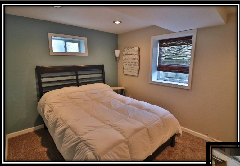
Bonus Room in Basement No Egress Window
