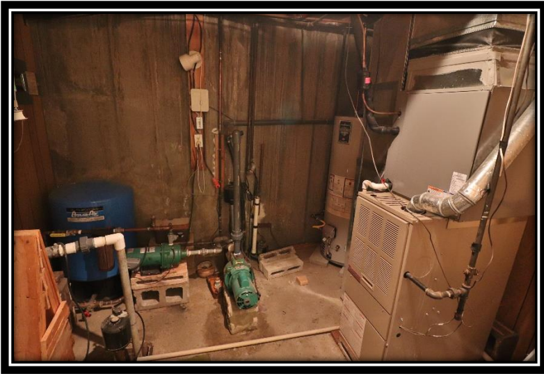
Utility Room in Basement
