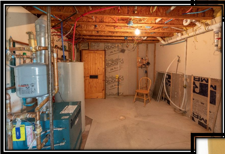
Storage in Basement
