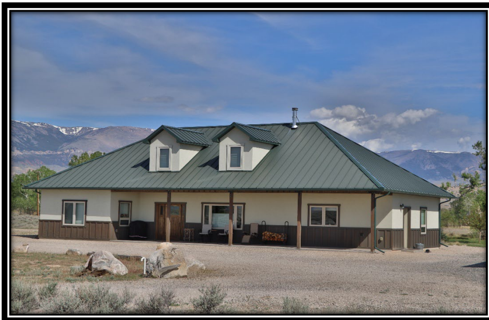
Clark Wyoming Home With Creek Frontage
