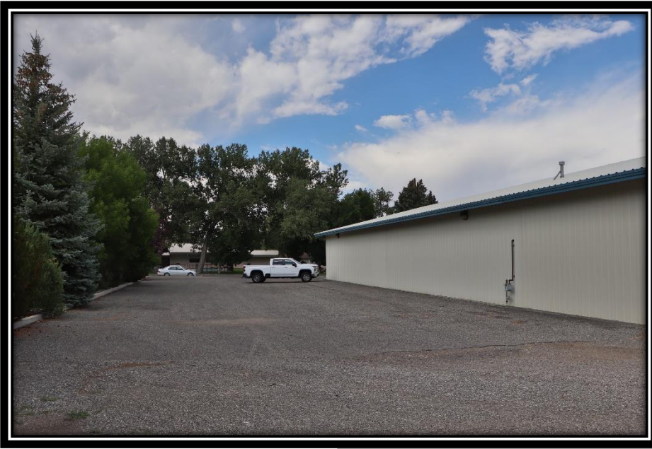
West Side of Building Looking North
