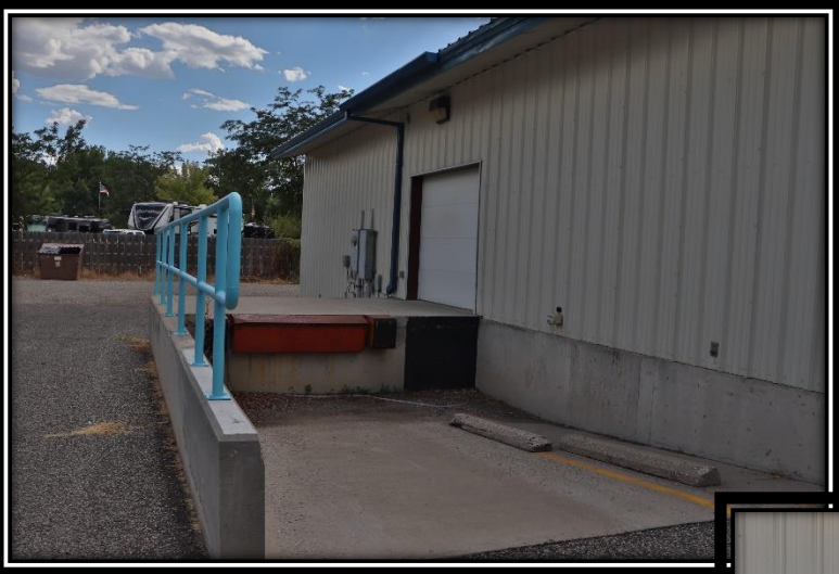
Loading/Unloading Dock On East Side
