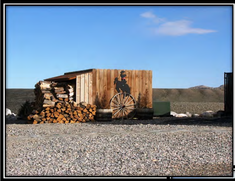
Shed for Propane Tank
